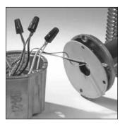
4. white-to-common, blackto-voltage. Screw on Junction box cover, making sure gasket is securely in place.
