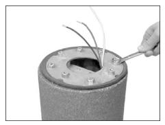
8 Insert mounting plate/driver assembly into concrete shaft. Center and align gasket and mounting plate on screw holes in concrete shaft. Tighten (4) 3/8" hex screws using a 9/16"wrench.
