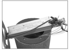
7. Place gasket on top of concrete shaft. Make connections between mounting plate/driver assembly and field wires, i.e. green-to-ground, white-to-common and black to voltage.
