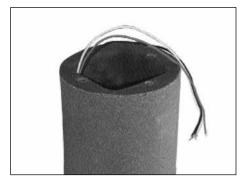
3. Route field wires through and out of top of bollard. Cocrete bollards are heavy; use adequate means to lift bollard and set onto anchor bolts without dropping. Install flat washers and 1/2" nuts.
