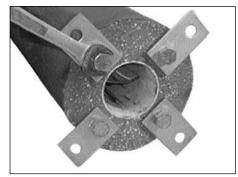
Install four anchor plates using 15/16" wrench with four 5/8-11 hex head bolts povided. Position the anchor plates straight from center on round bollards (see plan view below).
