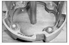
1. Install the base casting on the preset anchor bolts. Use flat washers and hex nuts both below and above the base casting.
