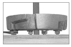
2. Level the top edge of the casting by adjusting the bottom leveling nuts. Tighten the upper nuts.
