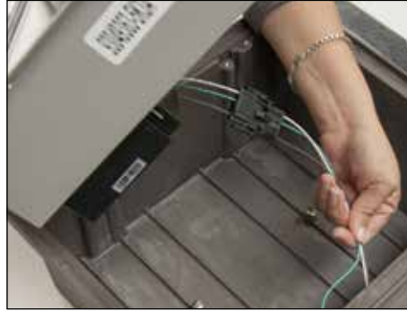
8. Begin installation of LED upgrade by connecting electronic driver wiring to line voltage
