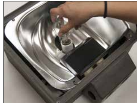
3. Unscrew and remove HID lamp.
