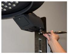
2. Tighten (4) bolts with 9/16" socket and ratchet on the adjustable die-cast plate at bottom of slip-fitter arm to secure the luminaire.
