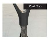
**4.** Use 9/16 socket with extension, expand the spreader to secure the fixture to the pole, torque to 20 lbs.
