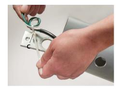
2. Lay pole horizontal on padded supports to protect finish. Pull field wires through pole and secure them with the tie-wrap (C) at the top of pole backing plate.
