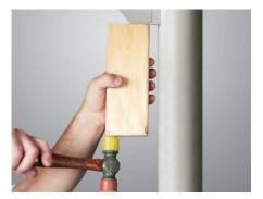
**2.** Place a wood block at base of luminaire arm and use a mallet to loosen fixture from Speed Mount.
