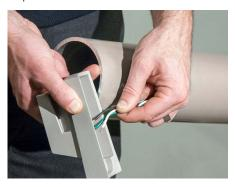
4. Pull wiring through speed mount. Make sure the wiring is long enough to reach terminal block on luminaire.
