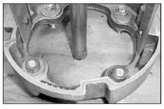
1. Install the base casting on the preset anchor bolts. Use flat washers and hex nuts both below and above the base casting.
