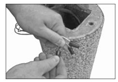
**8.** Make connections between driver assembly and field wires, i.e. greento-ground, white-to-common and black to voltage.
