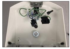
Remove all components from driver compartment including existing tray, leaving only incoming wire connections.
