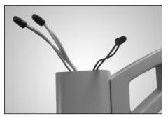
**4.** Connect fixture wires to field wires observing polarity, i.e.; green-to-ground, white-to-common and black-to-voltage.
