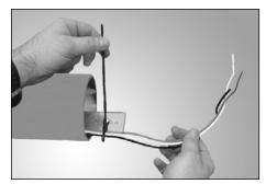
Lay pole horizontal on padded supports to protect finish. Pull field wires through pole and out the top. Tiewrap wires to pole backing plate. Tie wires in a knot or back loop through tie-wrap.
