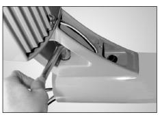
Attach fixture assembly to pole (2 places) using washer and C " bolt. Be sure fixture is aligned with anchor base and other fixtures for multiple mounts. Tighten to 20 ft.-lbs. using N" socket wrench.
