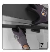
Put in lens latches. Repeat this step for continuous run. Ensure that the lens latches are fully engaged. An audible click will be heard when each latch spring locks and the bottom edge will sit flush with the external housing's edge
