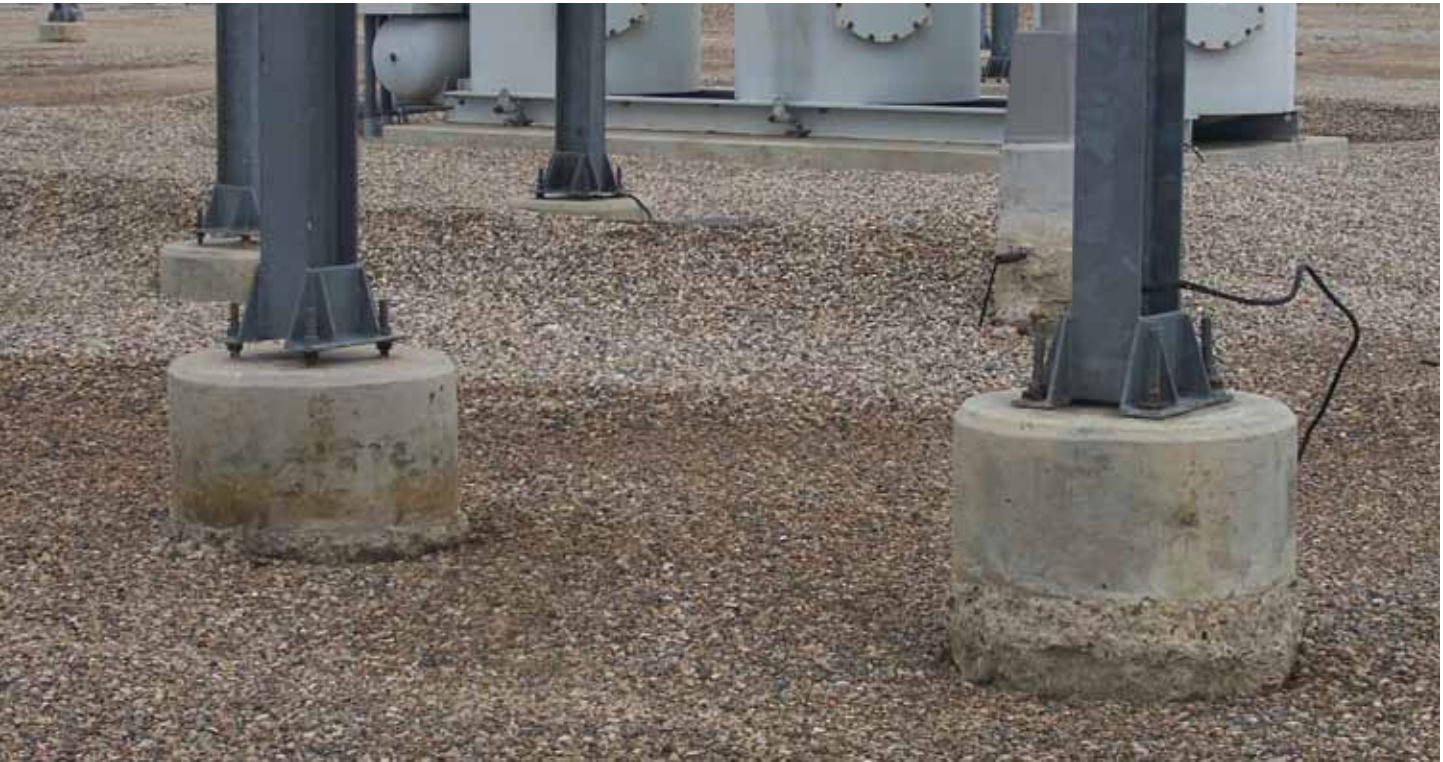
Frost heave created major problems at Basin Electric Cooperative's Logan substation. Concrete piers were 6 inches to 2 feet out of the ground. Notice the frost heave particularly evident on the pier at right, above.
