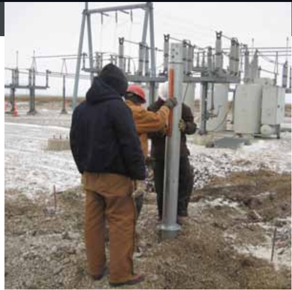
First, spotting the precise location for a Helical Pile’s lead section, then the drive tools engage the box coupler at its top.
