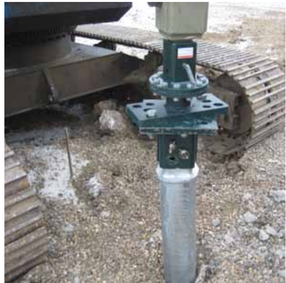
When the lead section is torqued into the ground, the Helical Pile’s baseplate section is added by bolting together their box couplers.
