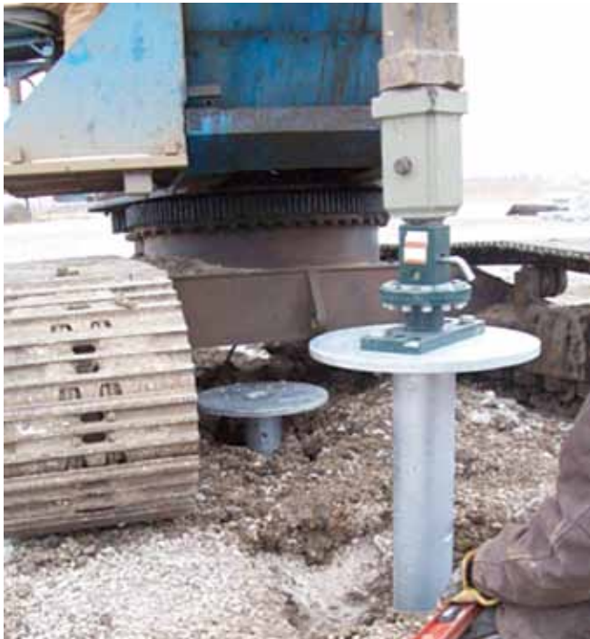
When the lead section is torqued into the ground, the Helical Pile’s baseplate section is added by bolting together their box couplers.
