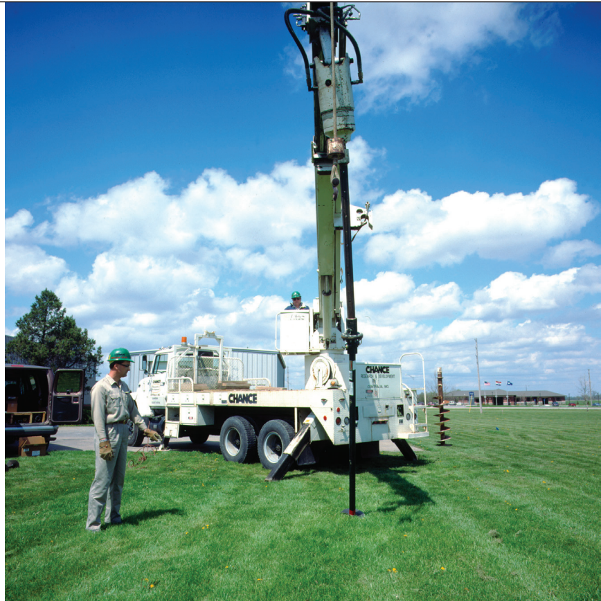
Operator and groundworker working together are critical to a successful anchor installation. PISA® 4 anchor shown below.
