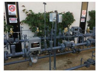
When an alarm from the pressure monitor is sensed, the associated transmission unit automatically switches to trend mode, sending live pressure reads to the utility every six minutes. When troubleshooting a fault, the utility also can remotely initiate trend mode on nearby transmission units for triangulation during alarm situations. The utility resets transmission units remotely once a problem is resolved.
