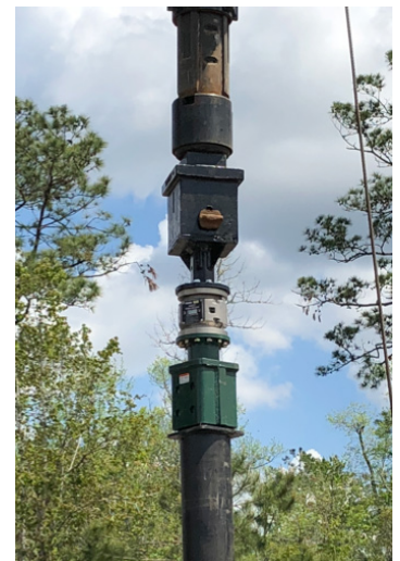
Fig. 3 Installation of the foundations monitored by a CHANCE® wireless torque indicator.
