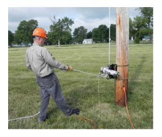
When the load is near the final point, slow down on the fall line pull to ease the load into position. With minimal practice, the operator can place the load within a fraction of an inch. Once the load is in place, lifting the foot from the control stops the hoist.
