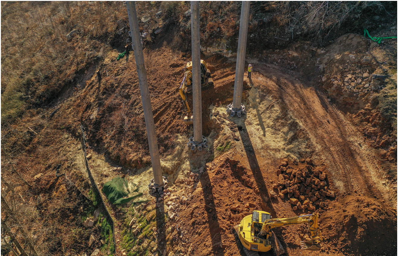
Structural framework designs for pole foundations are often used in areas with soft soil, which offers low load-bearing capacity. One or more tiers of wood or steel beams are connected to distribute the load over a wider area. Connecting micropiles to a grillage is not a common strategy. However, it can serve as a workable solution for mountainside locations. Photo by Hubbell.
