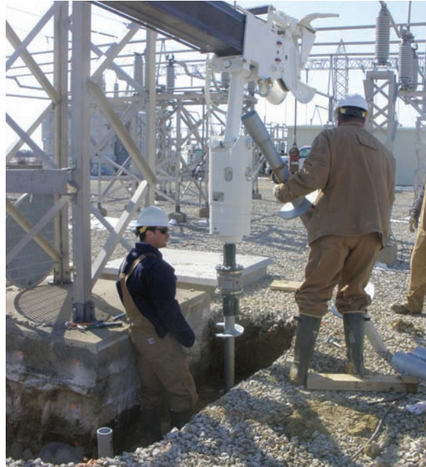
A work crew installs helical piles around three sides of an existing foundation.
