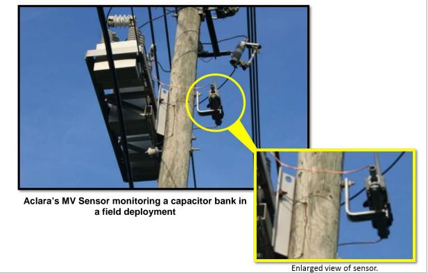
Above is a photograph of the full installation. Aclara's sensor is installed on the opposite side of the pole from the capacitor, utilizing the bracket seen above. The capacitor's neutral wire is then passed through the sensor to allow for current measurements..
