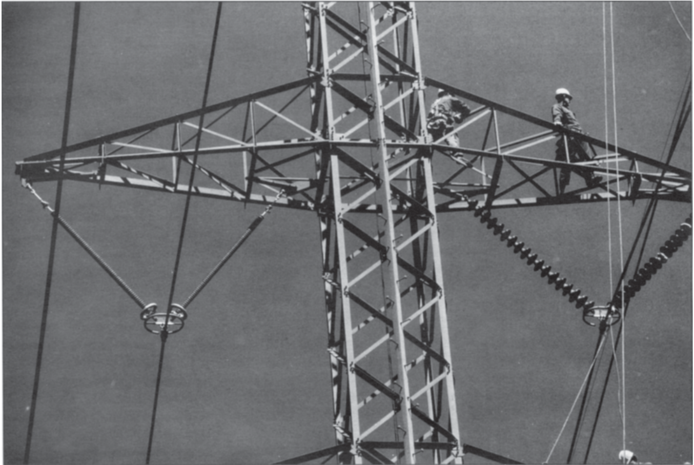
Linemen prefer working with lightweight polymer insulators.
