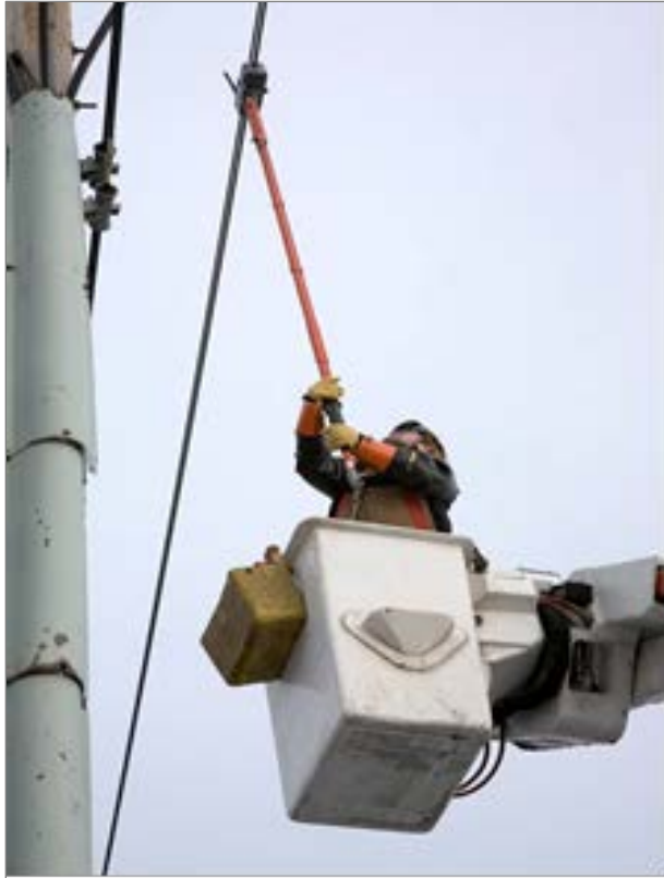
Figure 1: Hot stick installation
