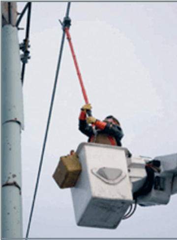
Figure 1: Hot-stick installation of Aclara's Sensors
