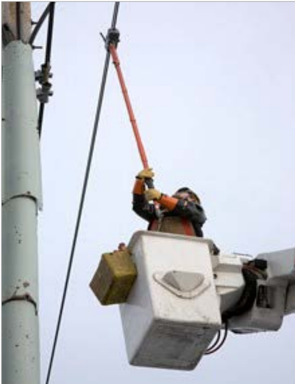
Smart Sensor Installation with Hot-Stick
