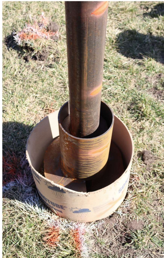
Photo 2: RS4500.337 x 8.63 OD Lead Section and Grout Reservoir
