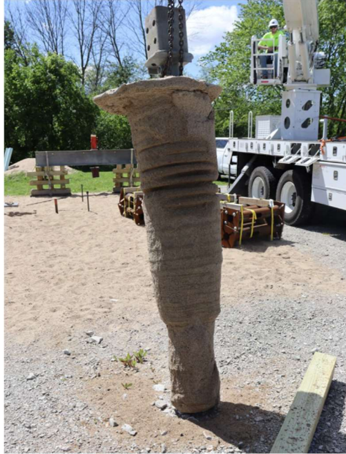
Photo 5: Excavated Tension Test Pile
