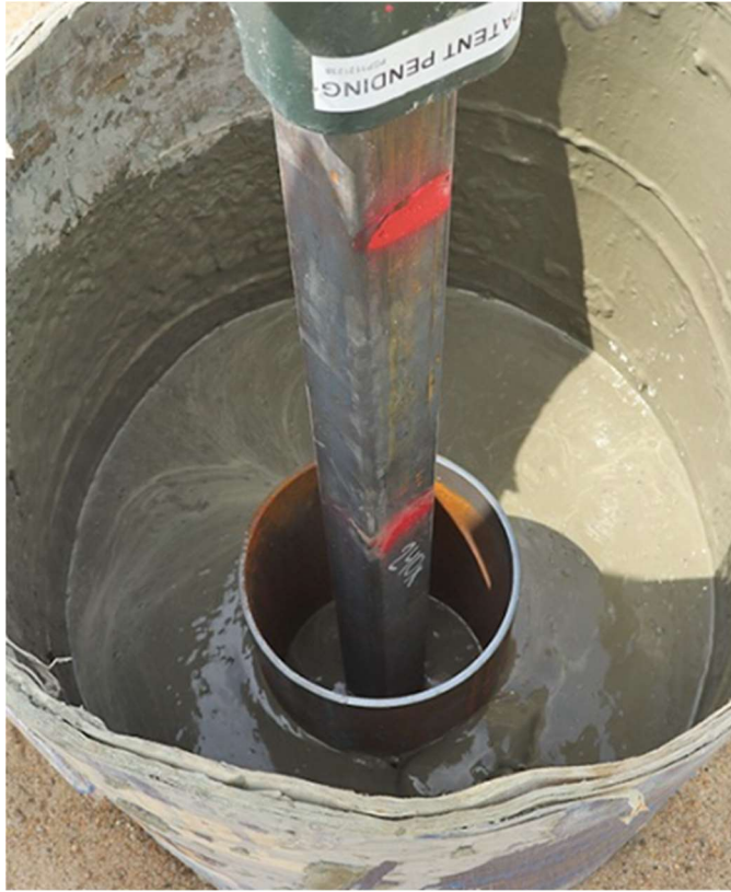
Photo 7: Installation of SS225 x 8.63 OD Test Pile
