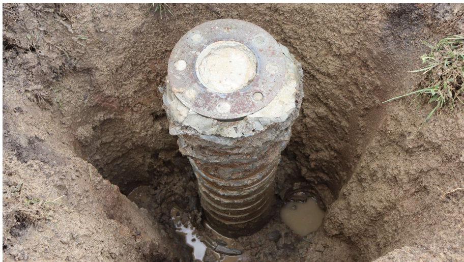
Photo 6: Excavated RS6625.280 x 12.75 OD Test Pile
