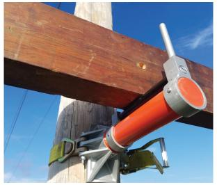
After removing DA Bolt, CCAT supports crossarm and facilitates movement into position to be lowered or installed.
