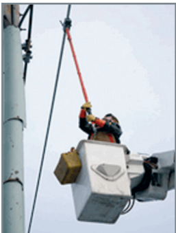
Figure 6: Aclara Smart Grid Sensor installation
