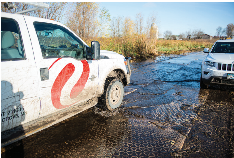
Matting was necessary to get vehicles and workers to almost all tower foundation sites.
