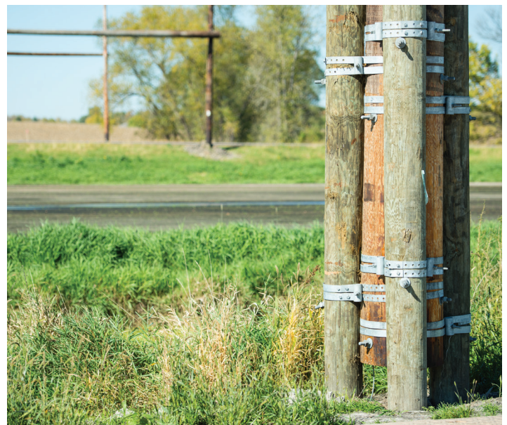
Xcel Energy had enough wood poles on hand to rebuild the first line, which was installed on driven wood pilings.
