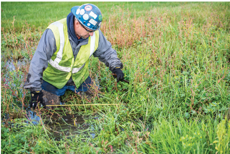
The engineering team determined where the tower would go, but the farmland and marsh terrain made the rebuild a challenge.
