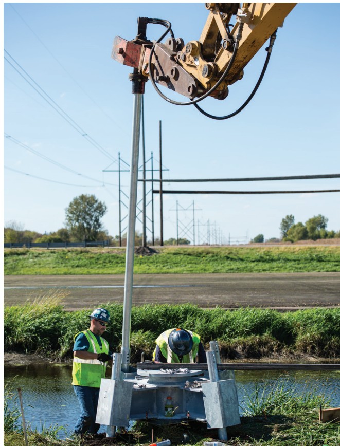
Helical piling supports the second steel pole line. These piles are installed with a drive head attached to a small digger and work well in poor load bearing soil, even marshland.
