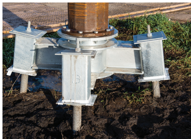
After the four permanent helical piles were drilled in, workers installed a grillage on top and grouted it in place. Then they installed a top cap and mounted the steel towers
