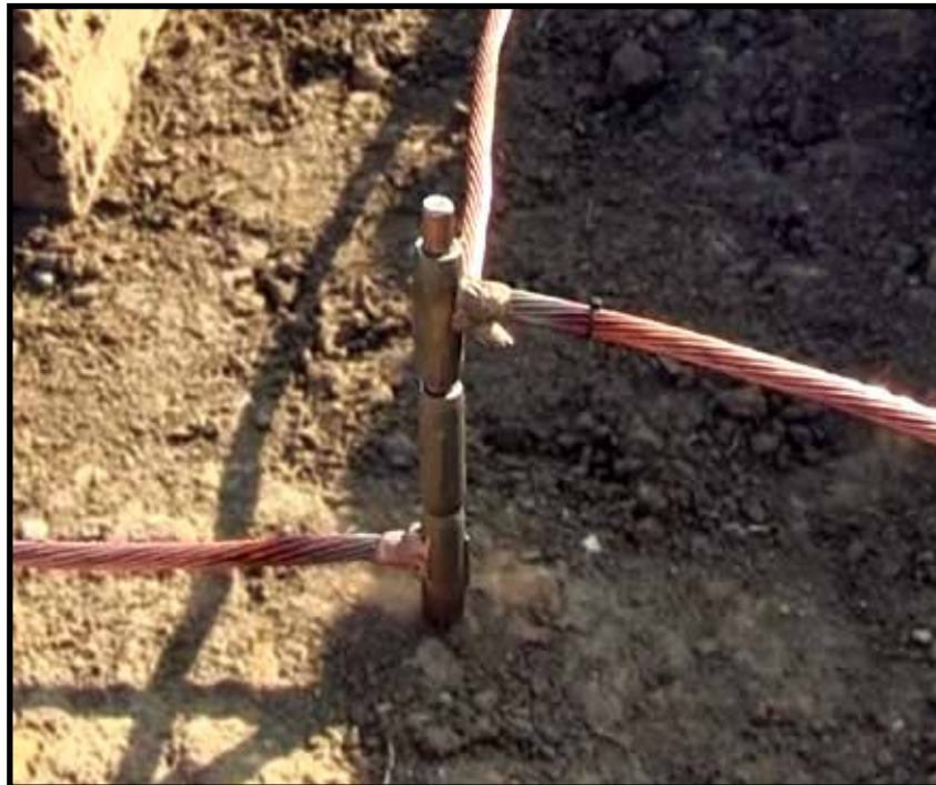
QuikTap™ stacked for multiple direction application.
