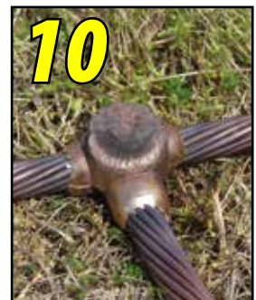
Remove weld and clean mold before making next connection.
