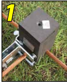
1 Position cleaned conductors in mold.
