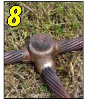
8 Remove weld and clean mold before making next connection.
