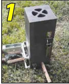
Position cleaned conductors in mold.
