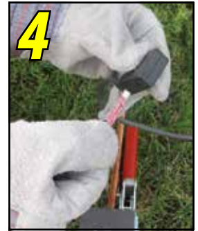
4 Insert the EZ Lite® Ignitor in the connector.
