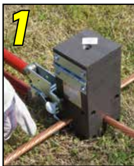
Position cleaned conductors in mold.
