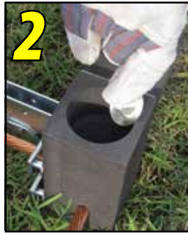
2 Place metal disc in bottom of mold crucible.
