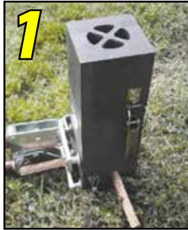
Position cleaned conductors in mold.
