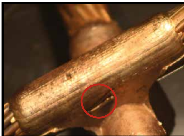
Image 7: Poor connectivity. Visible wire shown in weld.
