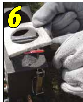
Place EZ Lite® Ignitor on the side of the mold and place gasket on top of ignitor.
