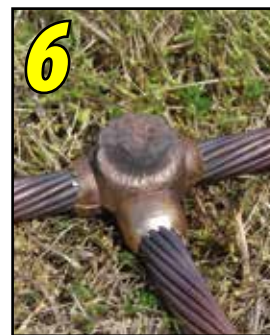
Remove weld and clean mold before making next connection.
