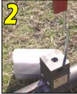
2 Position conductor and mold onto pipe.
