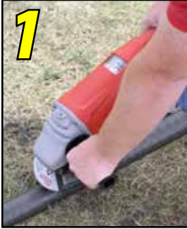
1 Clean pipe before making weld.
