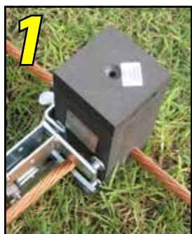
1 Position cleaned conductors in mold.
