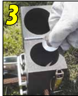
3 Place metal disc in bottom of mold crucible.
