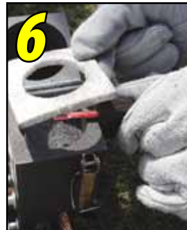
6 Place EZ Lite® Ignitor on the side of the mold and place gasket on top of ignitor.
