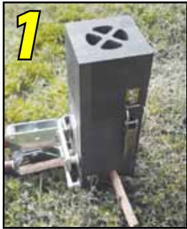
1 Position cleaned conductors in mold.
