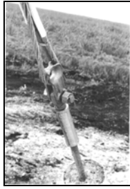
Fig. 1: Implosive sleeve connecting guy grip to steel anchor rod
