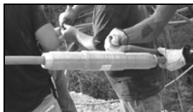
Fig. 2: Implosive splice ready for detonation
