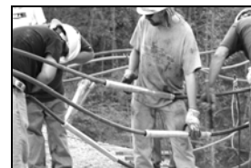
Fig. 5: Splicing crew preparing six implosive splices for simultaneous detonation
