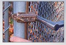
Manufactured from a high copper alloy, **BURNDY**° connectors are designed to last for the life of an electrical grounding system— 40 years or more.
