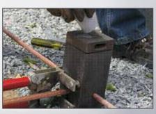
safety of the contained, high-temperature reaction; the irreversible connection; the lack of loosening or corrosion at the weld site; and no need for an outside power source.
