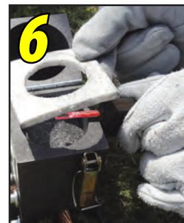
Place EZ Lite® Ignitor on side of the mold and place gasket on top of ignitor.
