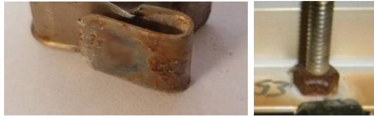
Figure 14: Corrosion of lower grade materials used in standard star washer connections
