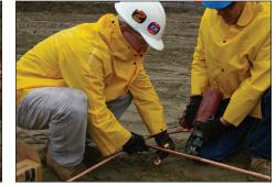
Our compression grounding system can be used for transformer grounding.
