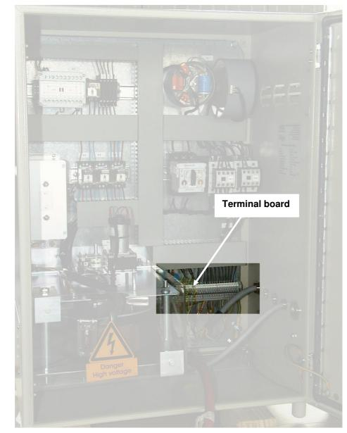
Fig. 55: Interior view of the STL 5 with terminal board
