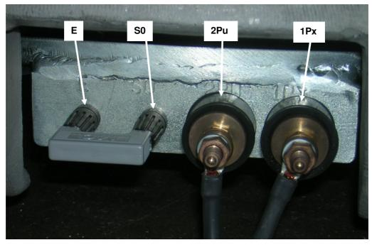
Fig. 60:Input terminals modulConnections without compensating reactors:
