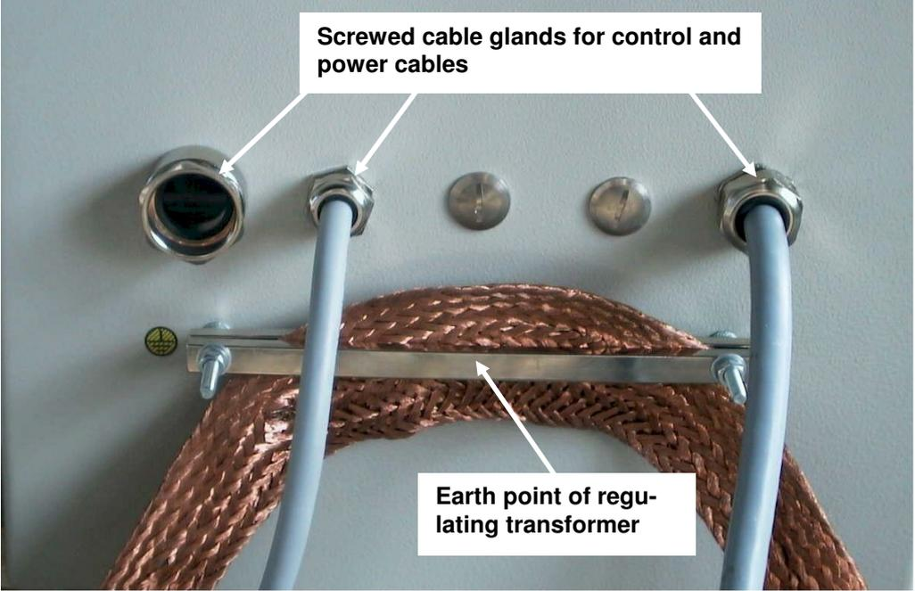
Fig. 57: Earth point of regulating transformer
