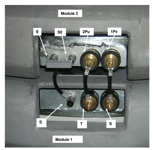
Fig. 61a: Connections between the two modules
