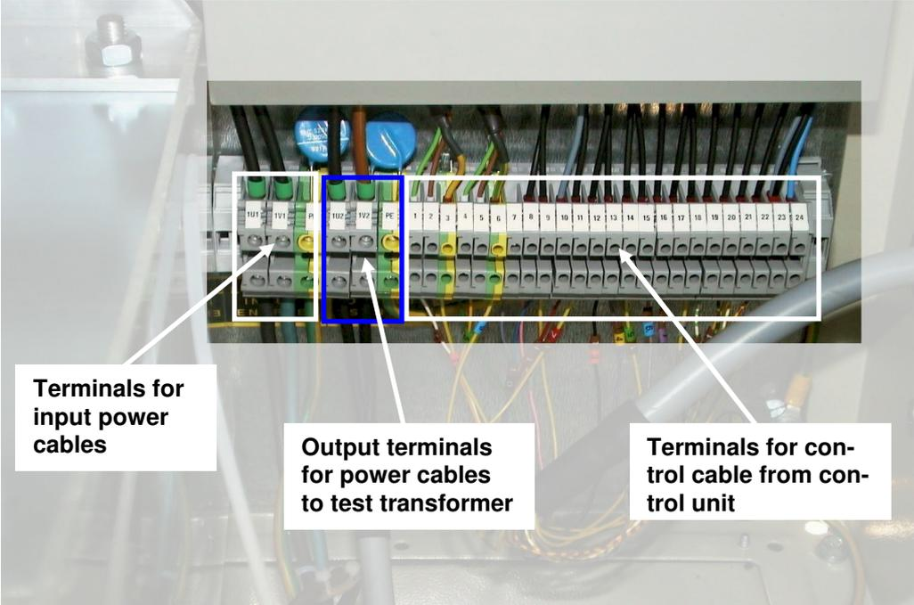
Fig. 56: Terminal board of regulating transformer
