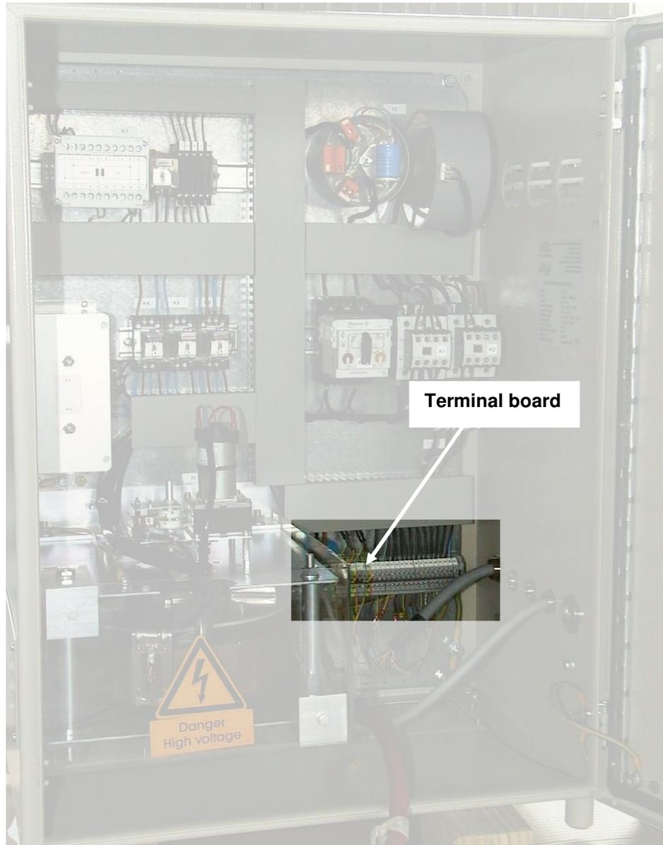
Fig. 55: Interior view of the STL 5 with terminal board
