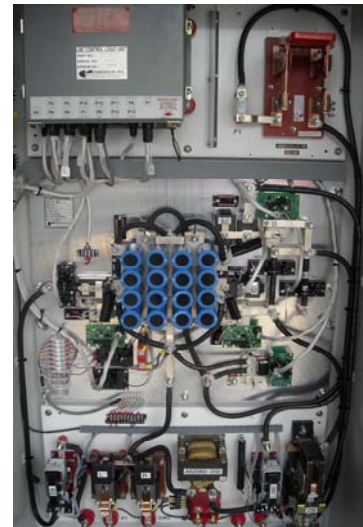
Typical Single-Motor Hoist Control Power Panel with Microprocessor Logic, 5-speed card & IGBT's
