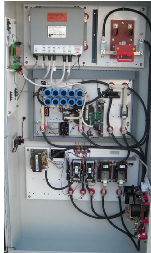
Typical Travel Drive--Logic, 5-Speed Card, IGBT Power Section and Contactor Panel
