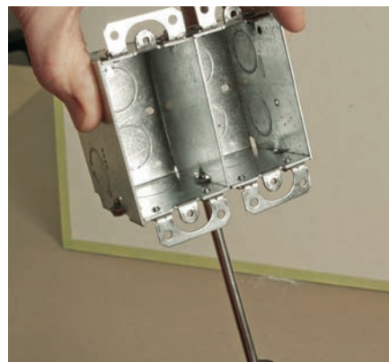
Step 4. Lock partition into position by tightening screws.
