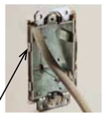
The plaster ears and GRIP-LOK® work together to hold the box in place
