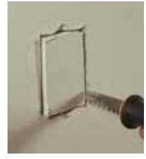
Cut an opening slightly larger than box size.
