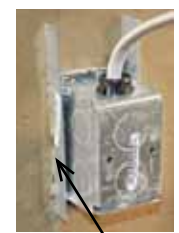
Keeping support snug against back of wall, fold tabs around front of box
