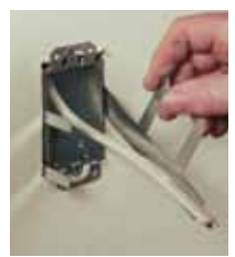
Insert a section of the GRIP-LOK® on both sides of the box
