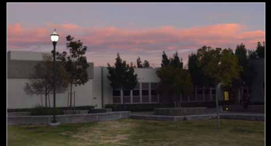
Job site – El Monte Highschool, El Monte, California
