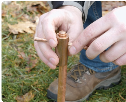
Insert conductor and place on ground rod
