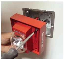
RACO® RETRO-RING® is used to position a 4" square steel box in an existing wall. RACO® 205RAC and 911-19 are used to support life safety appliance installations with or without boxes.\* \*can be used without a box when in compliance with local building codes
