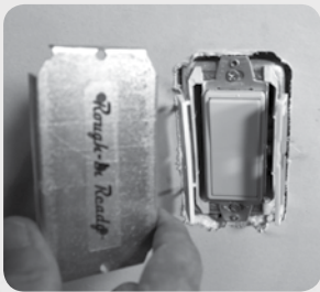
Remove Rough-in Ready® protection plate
