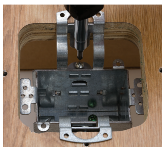
Mount & adjust box Install and wire device
