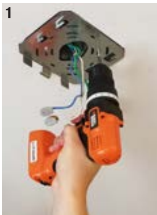
Mount plate to junction box.
