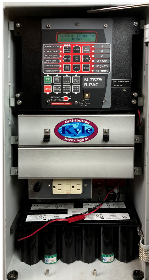
Figure 3 M-2406 Adapter Chassis Retrofit Completed
