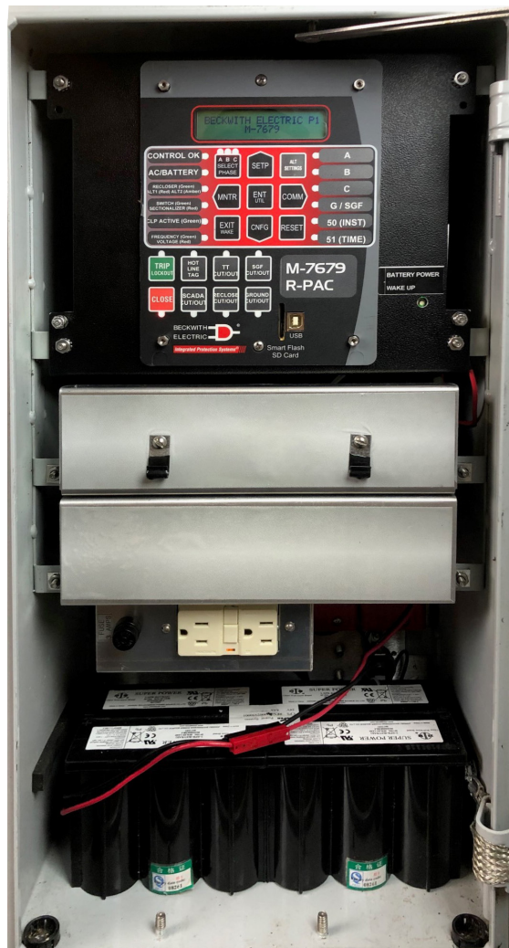
Figure 4 M-2406 Adapter Chassis Retrofit Completed
