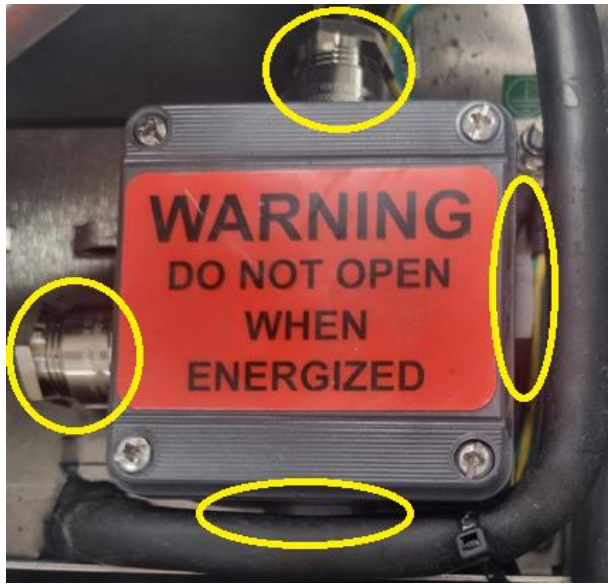
Figure 2. Austdac UPS internal Ex e enclosure
