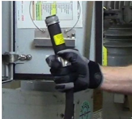
Figure 2 Disconnect 14-Pin or 19-Pin Recloser Cable
