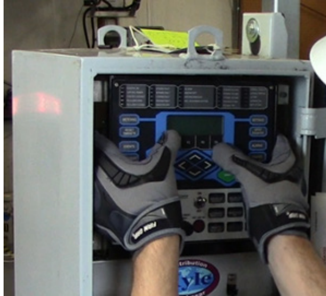
Figure 15 Removing the Eaton Cooper Control from the Cabinet
