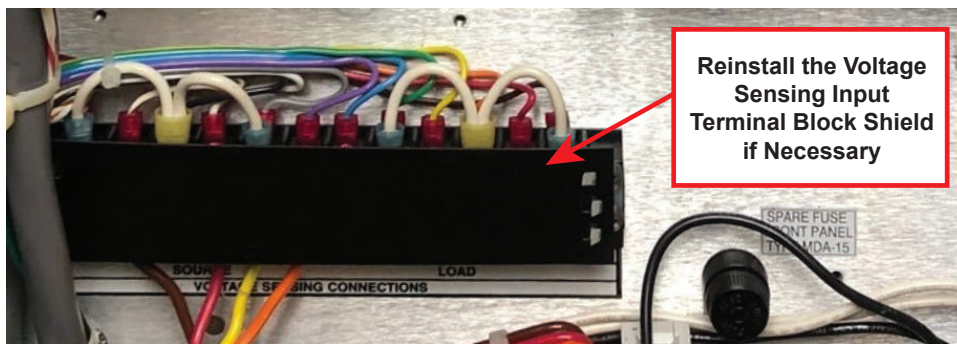
Figure 23 Optional Voltage Sensing Input Terminal Block Cover Shield
